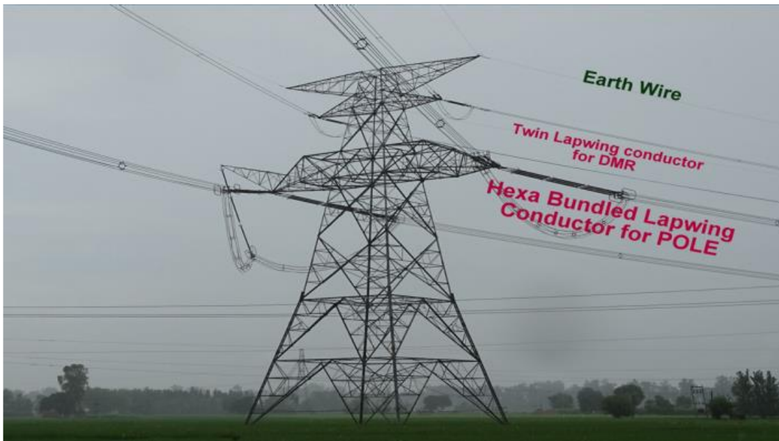
Figure 4-3 +/- 800 kV Tower For CK2 Project in India with Dedicated Metallic Return Conductor (DMR)
