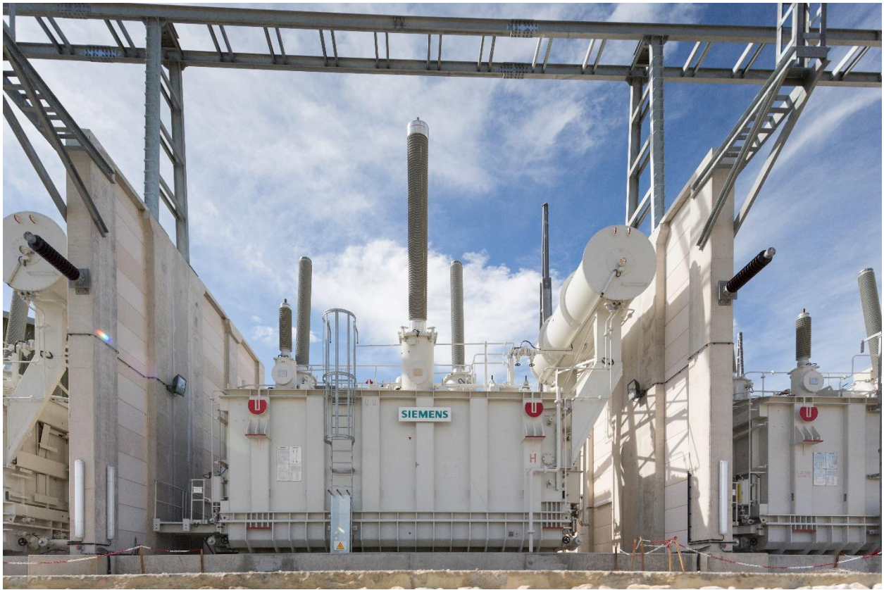
Figure 3-6 Converter Transformer
