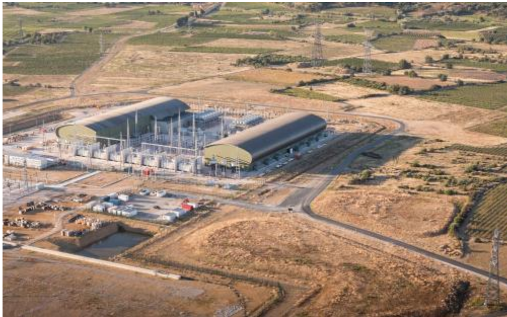
Figure 3-4 INELFE 2X1000 MW VSC symmetrical monopoles at Biexas France-Press release by Siemens
