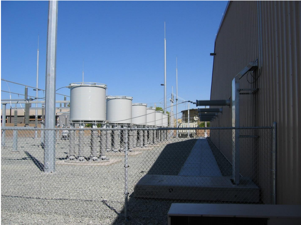
Figure 3-8 Phase reactors
