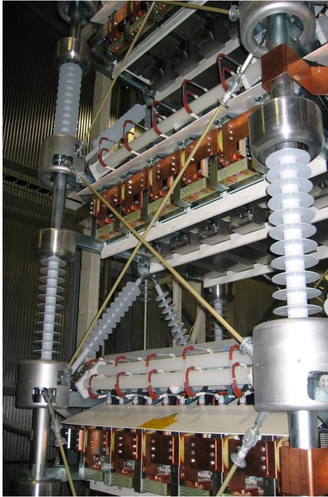
Figure 3-2 VSC converter valves courtesy of siemens
