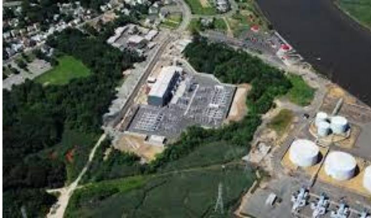
Figure 3-10 Neptune Regional transmission Sayreville substation USA
